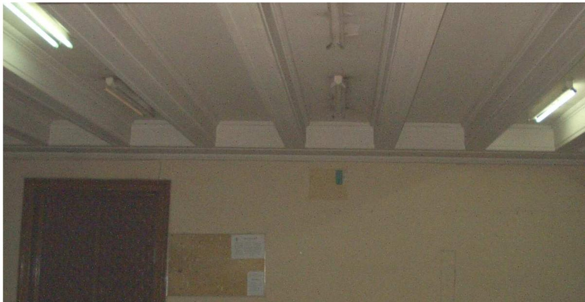
**Photography of buttresses (concrete girders) on the ceiling of 4-rd floor of the Physics Department measured with GPR**
