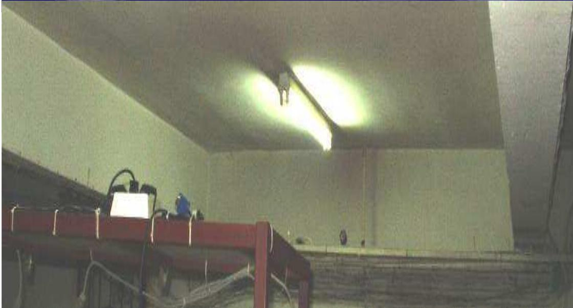
**Photography of the buttresses (concrete girders) on the ceiling of the basement of Building B of Physics Department measured with GPR (above).**
